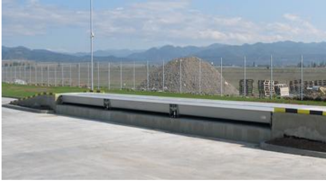
Scale shown above ground with concrete Ramps
